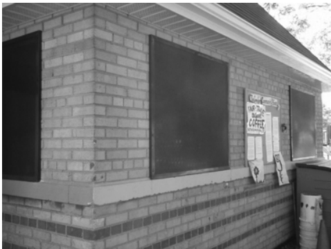
Front of Field House
