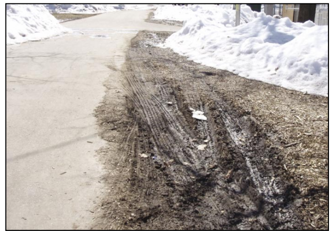
Deep ruts beside the asphalt path
