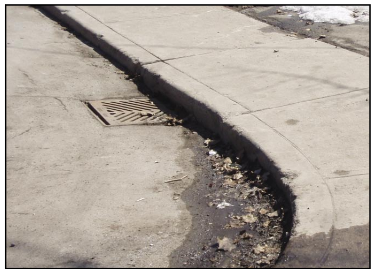
Detail of catch basin
