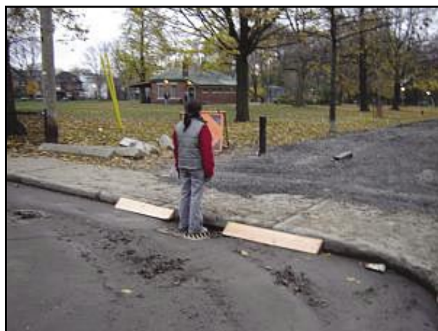
Wedges made by the carpentry shop
