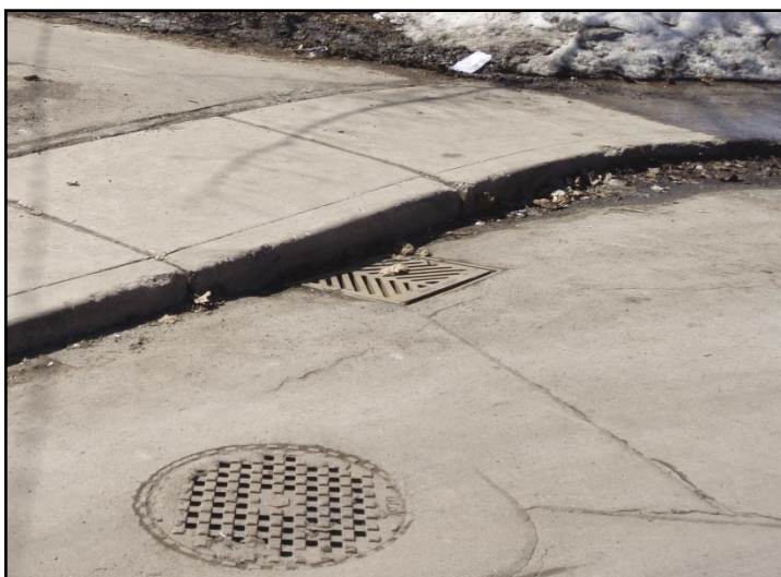
Detail of drainage
